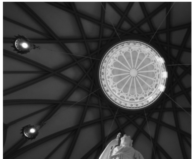
A view from the floor of the Main Library up into the dome
