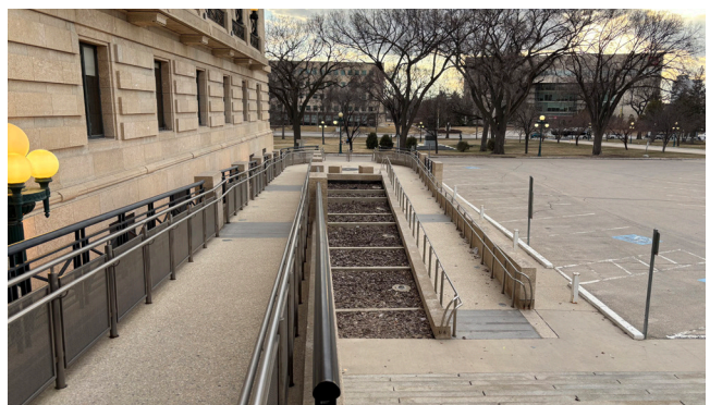
The Assembly's exterior wheelchair ramp.
